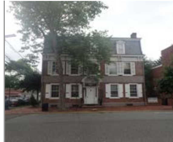
Francis Hopkinson House, Bordentown, Burlington County
