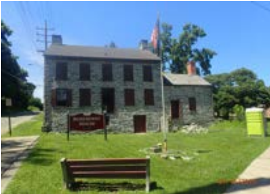
Roseberry House, Phillipsburg, Warren County
