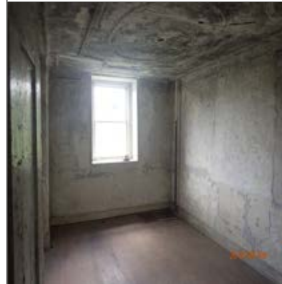
Interior of The 1759 Vought House with elaborate plaster ceiling, Clinton, Hunterdon County
