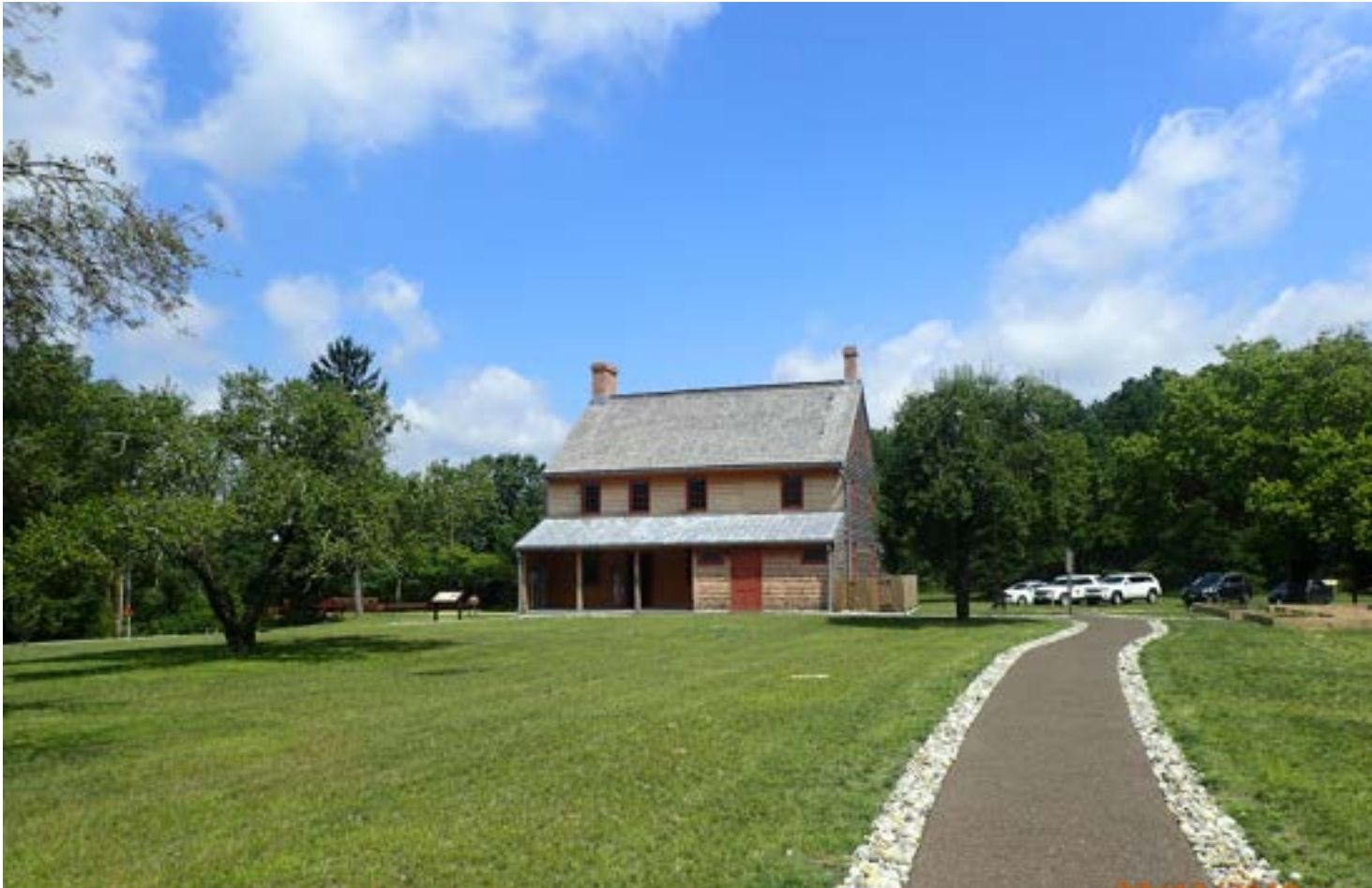
Cedar Bridge Tavern, Barnegat, Ocean County
