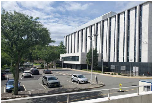
Rear of the State Archives Building; this is the location of a potential addition that could house a portion of the Experience Center (Site option 3)
