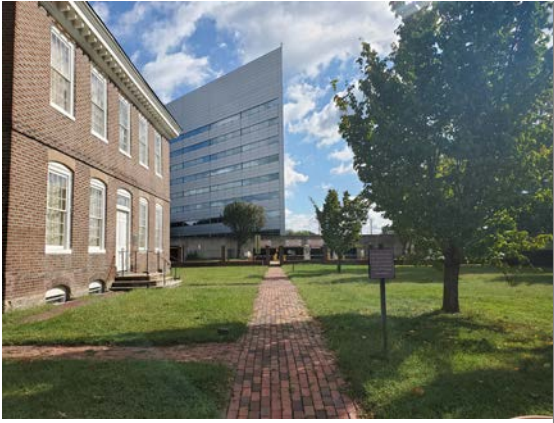
The main entry of the Trent House looking towards the N.J. Justice Complex
