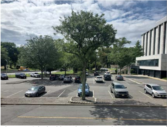
The rear of the building that houses the N.J. State Archives; Route 29 is to the left
